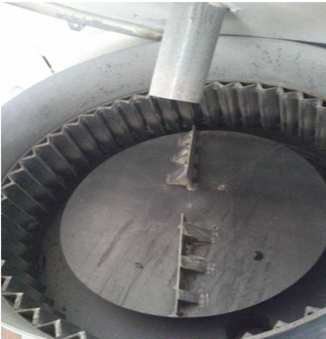
Fig. 2. Internal view of the crusher
